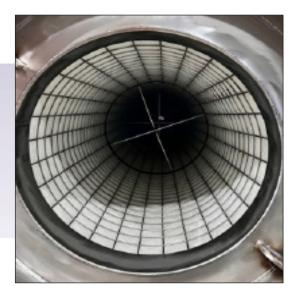
Atephos mist eliminators are capable of reaching an efficiency level of 99.5% for sub micron aerosols. For droplets over 1.5 microns, the efficiency is 100%.
